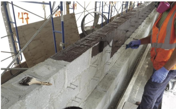
► A liquid-applied air barrier provides a continuous layer of moisture protection.
